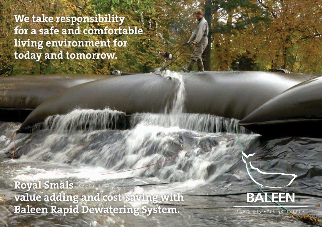
With geotextile containers the cost-saving process is signified. By dewatering the sludge, volumes can significantly be reduced by up to 50%. This innovative system is more efficient than all other classical sedimentations, and cheaper than mechanical dewatering processes.
