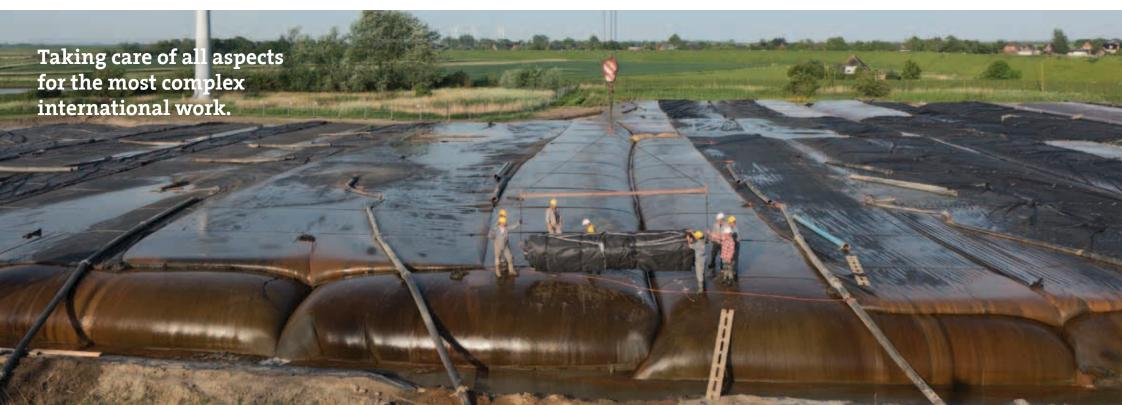
With Baleen RDS we present a significant added-value process. We can use the sediments in the ecological geotextile containers for new valuable constructions.
